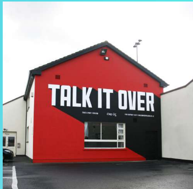
(Above) Eire Og Club House is one of Paul's most recognised works.
